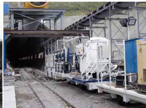
Austria, Wienerwald RAILWAY TUNNEL
